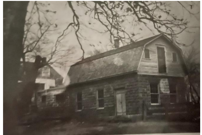
The plant was built around this building located on the Xavier and Elizabeth Hartrich Picquet estate.
