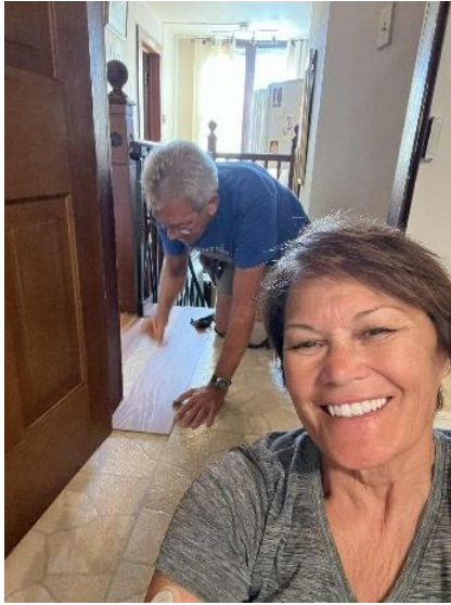
Larry and Dolores Hahn installing upstairs flooring
