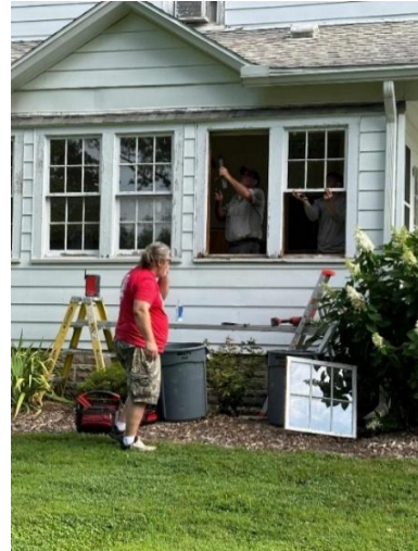
John Geltz crew installing new windows in sunroom
