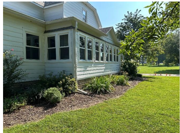
New Windows in Sun Room
